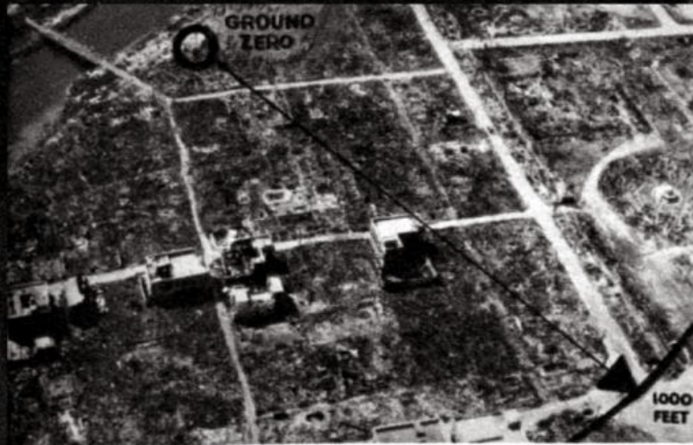
As close as 1,000 ft. from the A-blast center in Hiroshima, these "American-type" buildings were left standing. Razed areas were gutted by fire.
